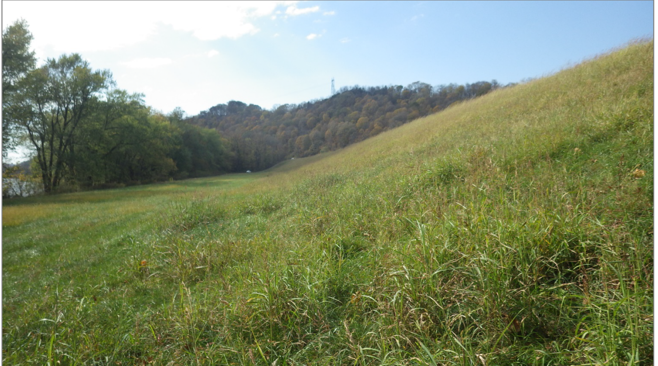
Photograph 5 – Southern dike embankment downstream side, looking west. Note tall grass.
