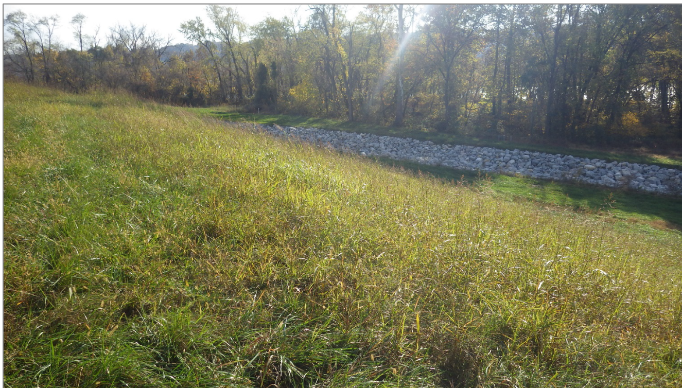
Photograph 6 – Western downstream side where the channel extends along the face and toe of the embankment. Note tall grass along slope.
