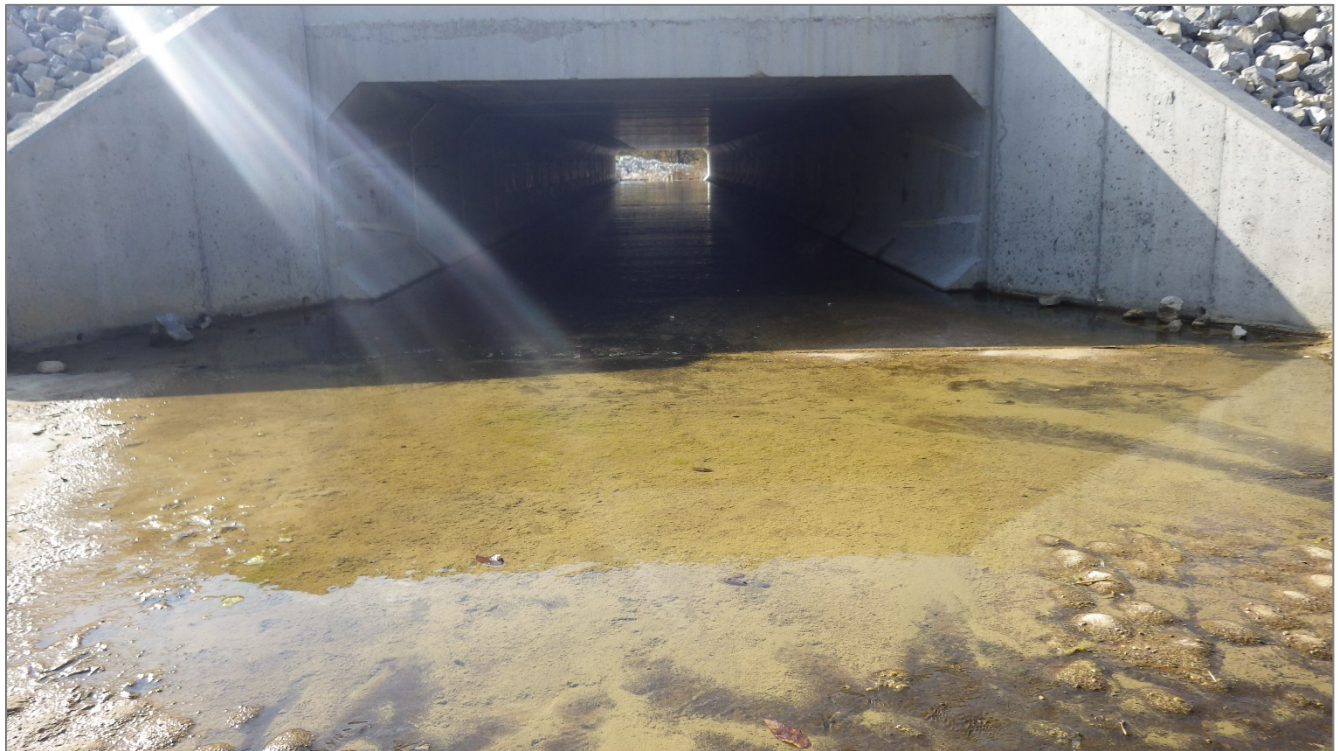
Photograph 11 – Upstream side of dam at 12 ft. x 4 ft. culvert, looking southwest through the culvert.
