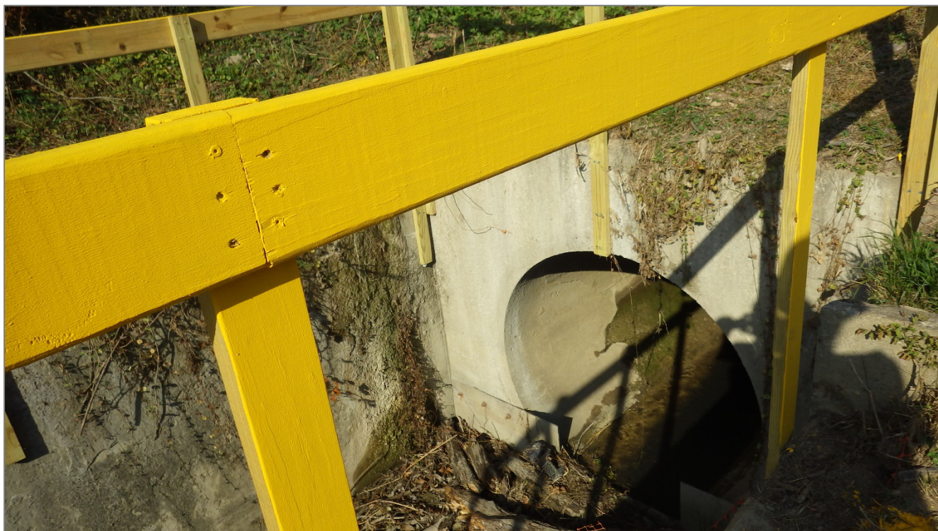
Photograph 5 – Outfall 001 outlet structure at toe of dam.
