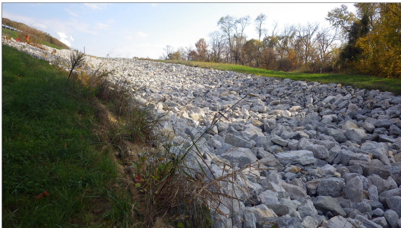
Photograph 4 – Western downstream channel showing erosion due to material change and silt fence removal.
